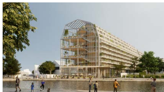
Aubervilliers, Coliving, coworking, restaurant, salle de sport
